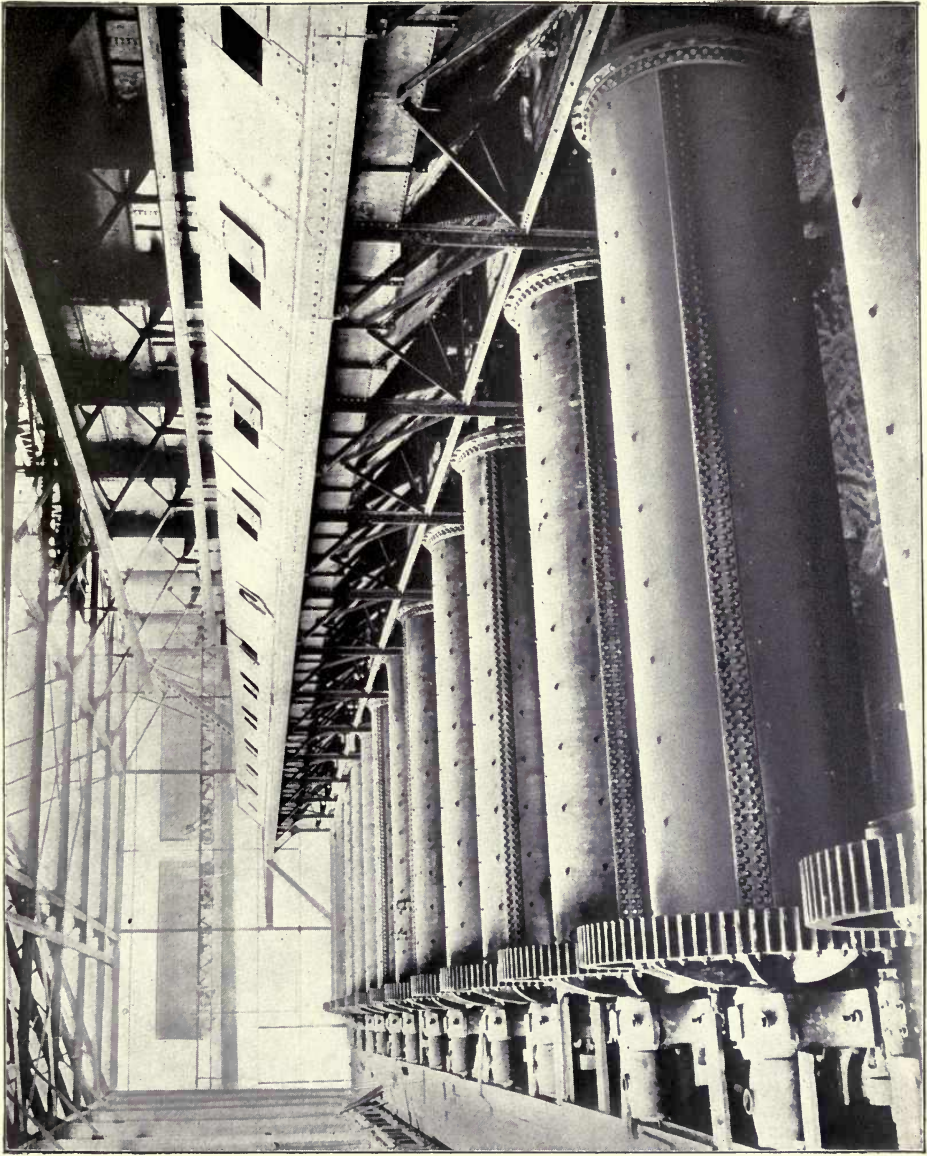
Tube mill installation. (Allis-Chalmers Co.)
